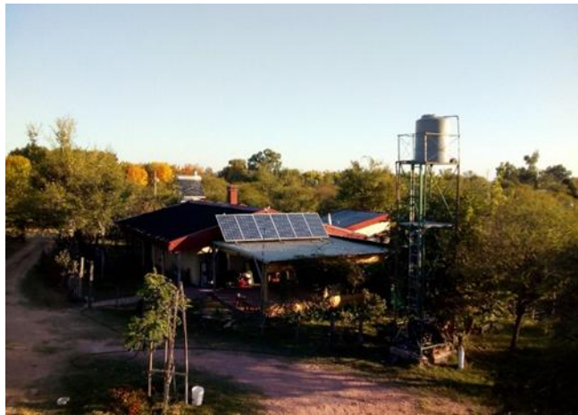
Figure 6. View of the house
